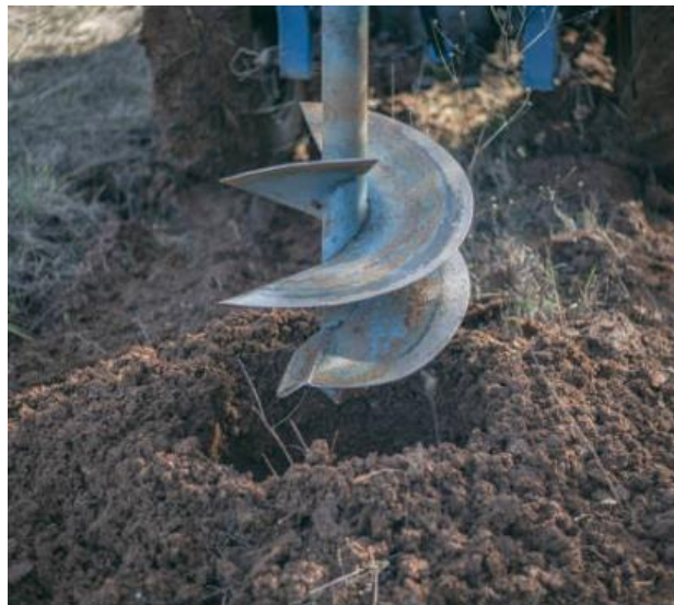
Auger drill for pole install
